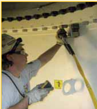
▲ Tightening tower segments.
