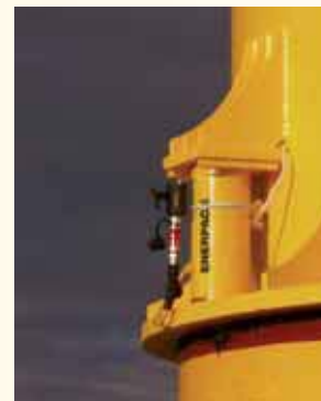
▲ Precisely leveling and positioning of off-shore wind turbine foundations. This 430-ton tri-pile foundation was levelled with three hydraulic cylinders mounted in each pile and using the PLC-controlled synchronous system. Precision to 0.04 inch (1,0mm) can be obtained.
