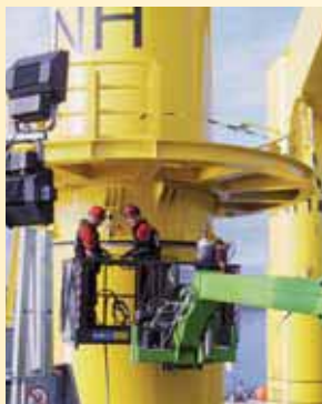
▲ Precisely leveling and positioning of off-shore wind turbine foundations. This 430-ton tri-pile foundation was levelled with three hydraulic cylinders mounted in each pile and using the PLC-controlled synchronous system. Precision to 0.04 inch (1,0mm) can be obtained.
