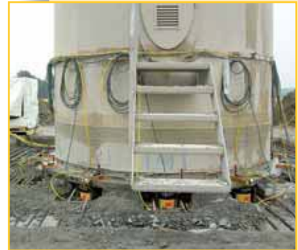
Realigning turbine foundation ▼
